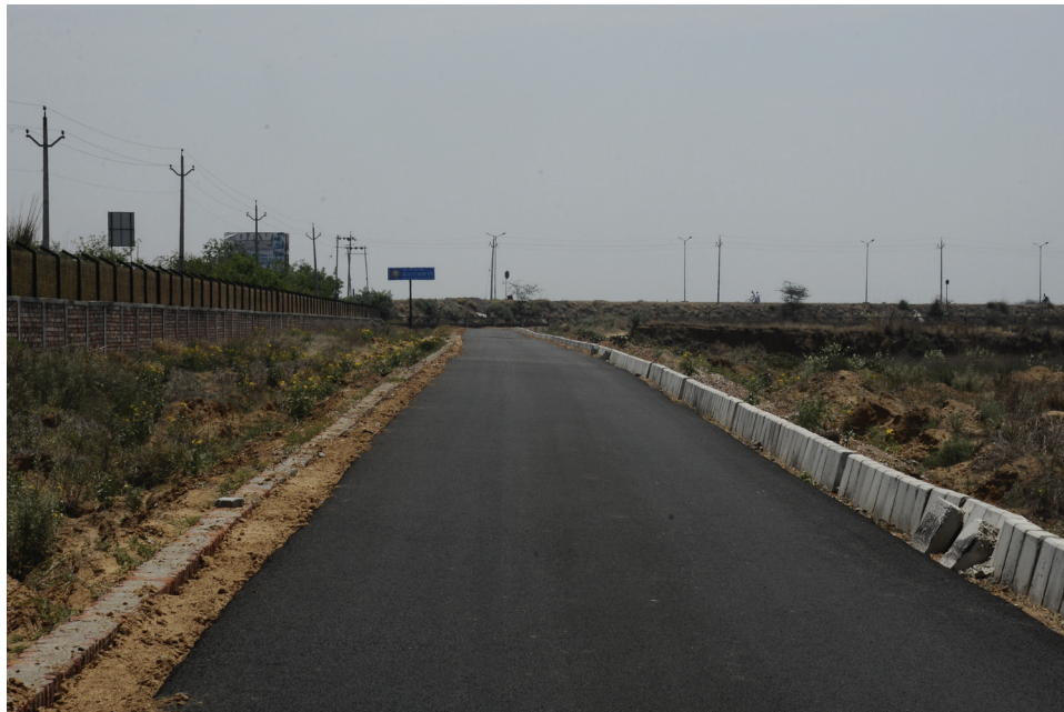
Internal Perimeter Road
